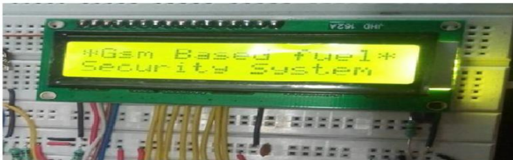
After switching on the system, the GSM based fuel theft security is installed.
