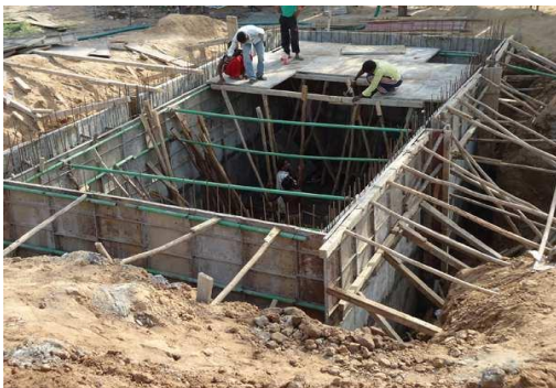
Fig 1 : Construction of Underground Reservoir
