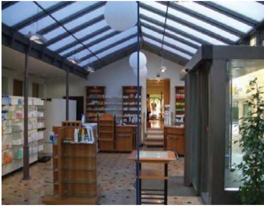
Fig. 4 : Translucent aerogel roof in a pharmacy of Switzerland
